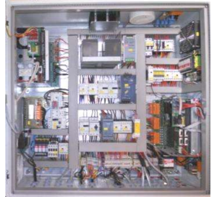
SETEC's wind-turbine control cabinet
